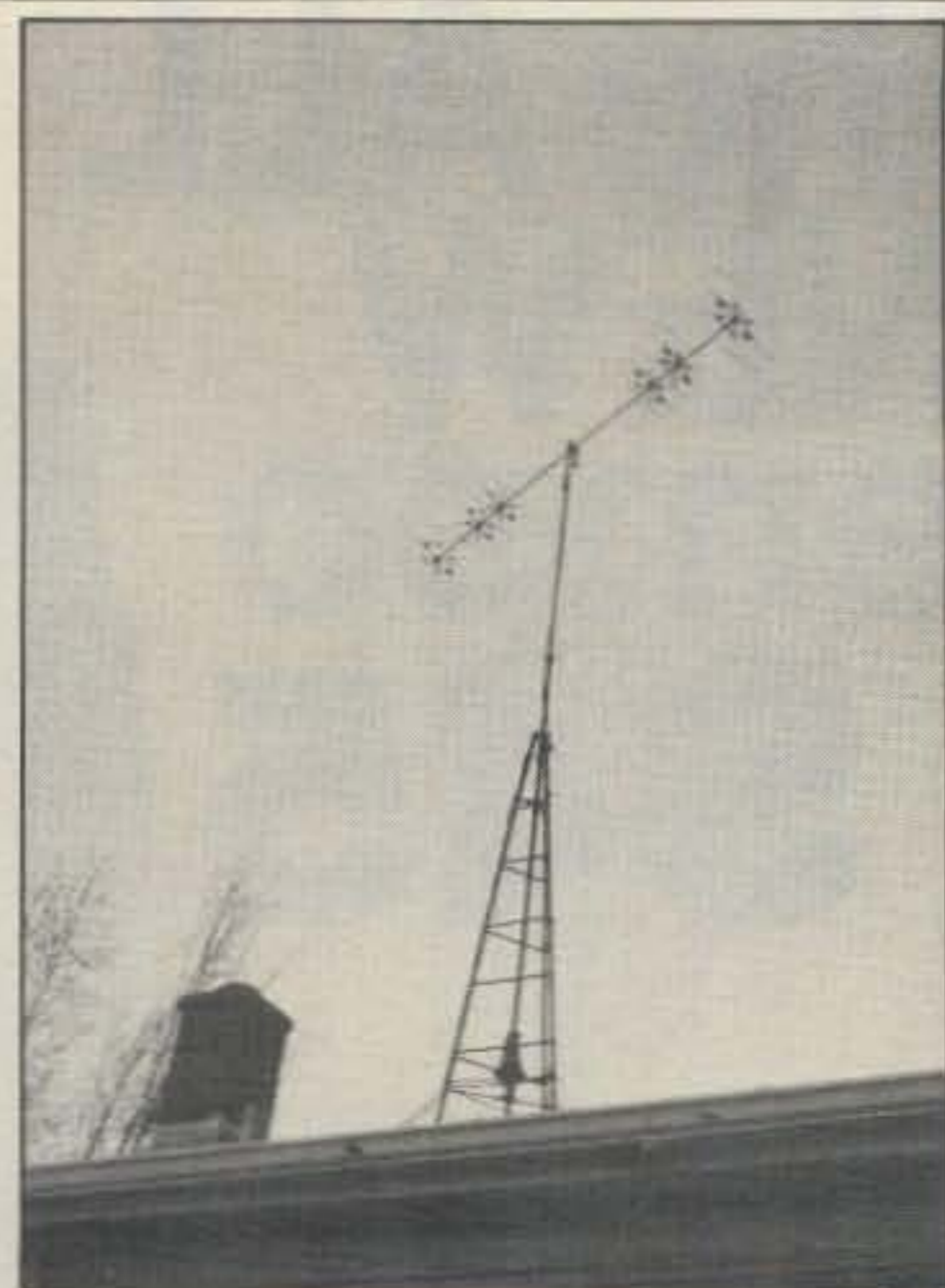
Fig. 6—The antenna is installed on a TV push-up mast mounted in a 10 foot tripod. The top of the tripod has been modified with a bearing and the entire mast rotates. The rotor is at roof-top level.
